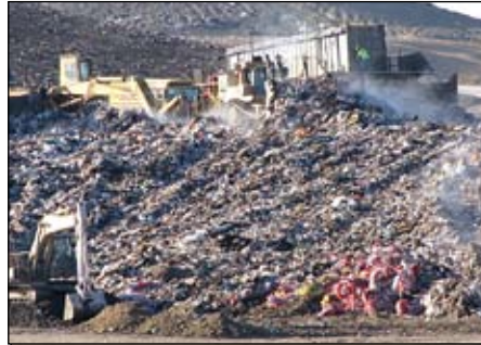
Photo left: Closeup of disposal site. Members process 7,500 tons of waste per day.
