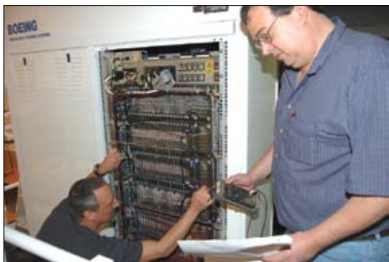
Pete Armstrong and Ray Ebach repair electronic panels on the KC-135 simulator.
