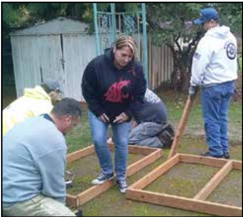
Machinists frame one of the two ramps for the Marysville resident.
