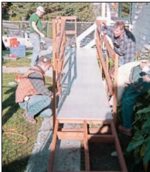
Volunteers put finishing touches on a wheelchair ramp.
