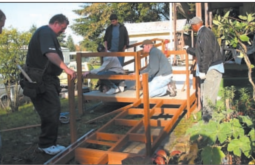
...member, members construct a wheelchair ramp for a Federal Way resident.
