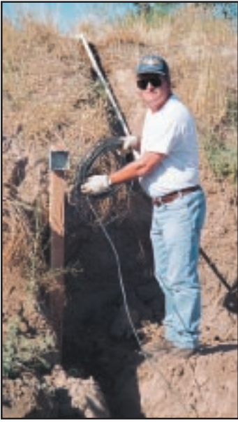
Photo left: Steve Reynolds runs control wire for a sprinkler system members repaired.
